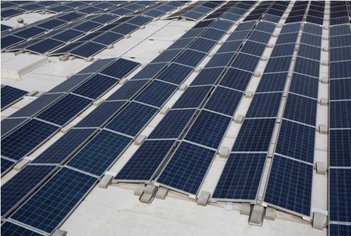
Figure 1 The solar farm is one of the largest in the city and is expected to generate 1.1 million kilowatt hours of power - enough to power 88 homes and reduce carbon dioxide emissions by about 1.4 million pounds annually. (ESTER SEGRETTO)
